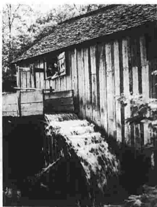
...and still drives the mill.
