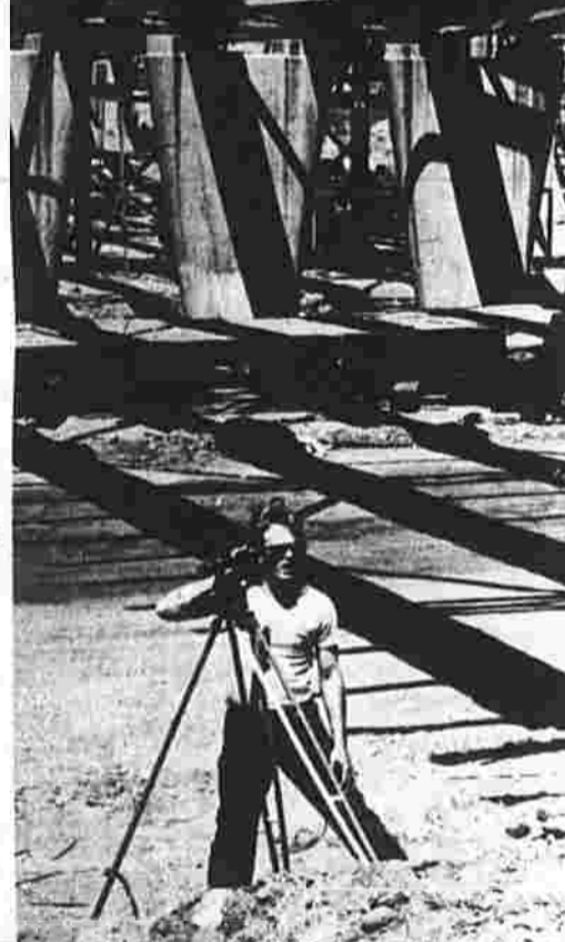
Steel girders and concrete stanchions dwarf a surveyor and his transit.
