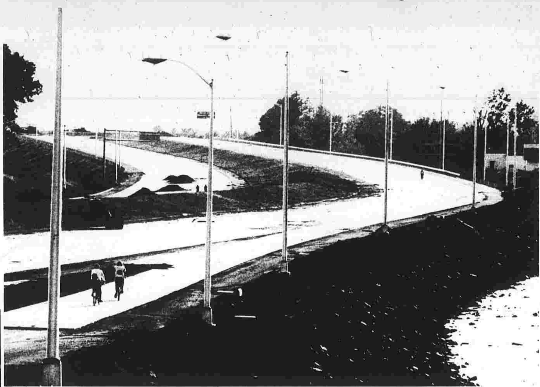
West of Keeney St., ribbons of concrete curving toward Hartford lure bicyclists on a twilight ride.
