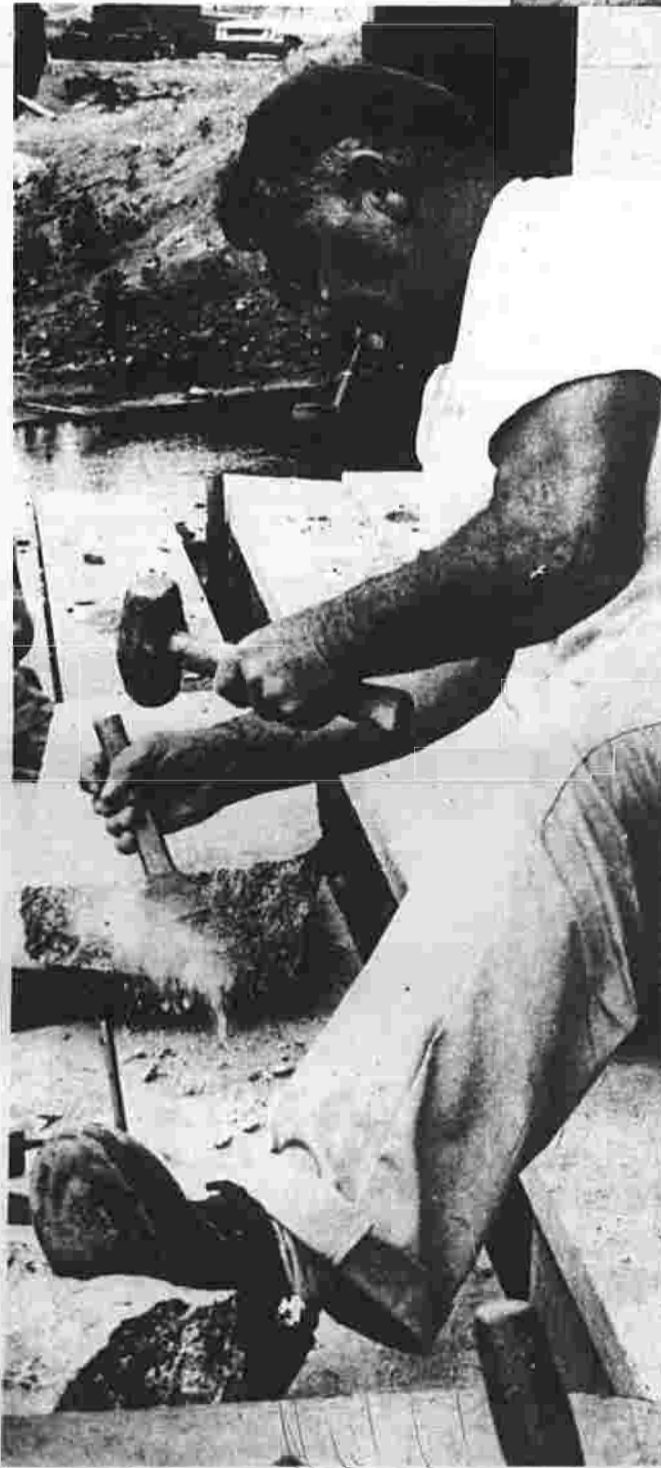
Pipe clenching a bridge on ramp where Gould's Pond used to be.
