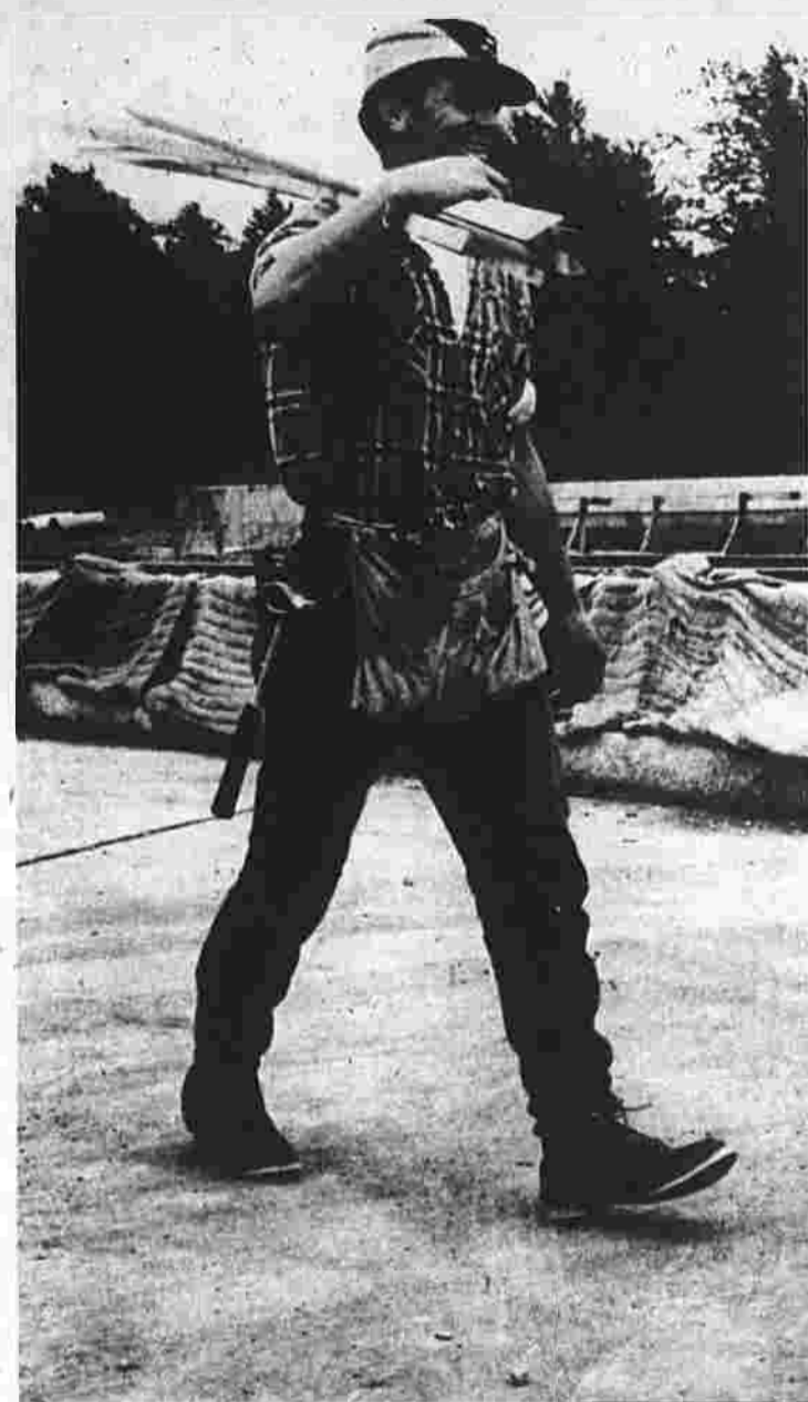
A carpenter builds forms for the Main—S. Main Sts. bridge abutment.
